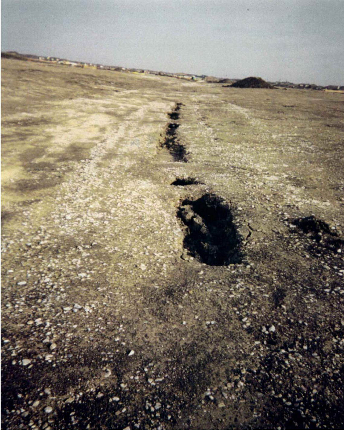
Photograph 1. Collapse of utility ditch backfill.
