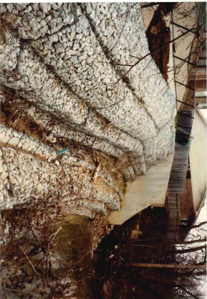
Photograph 8. Condition of east end of gabion wall after 1991 flood.
