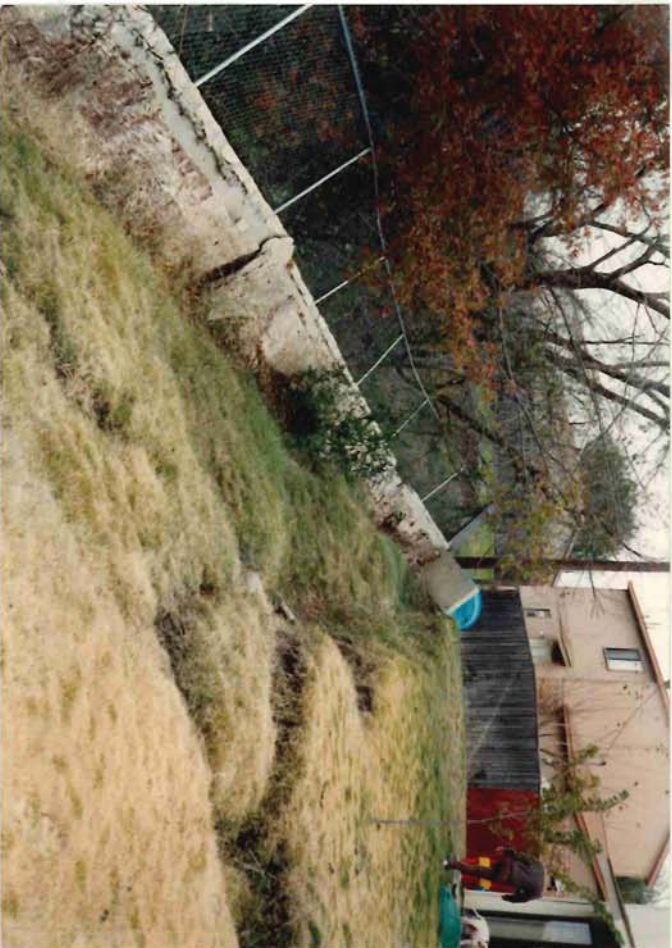
Photograph 12. Head scarp of slope failure at 413 Brandon Street.
