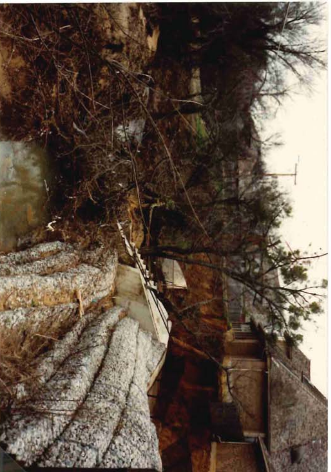
Photograph 7. Condition of gabion wall after November 1991 flood. Camera pointed west. Residence on Lot A is located in the upper right corner of the photograph.
