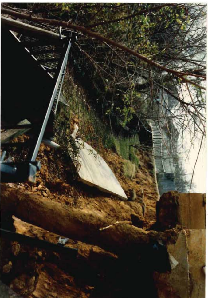
Photograph 9. Head scarp on Lot A. Portion of foundation on Lot A is visible on the right side of photograph.
