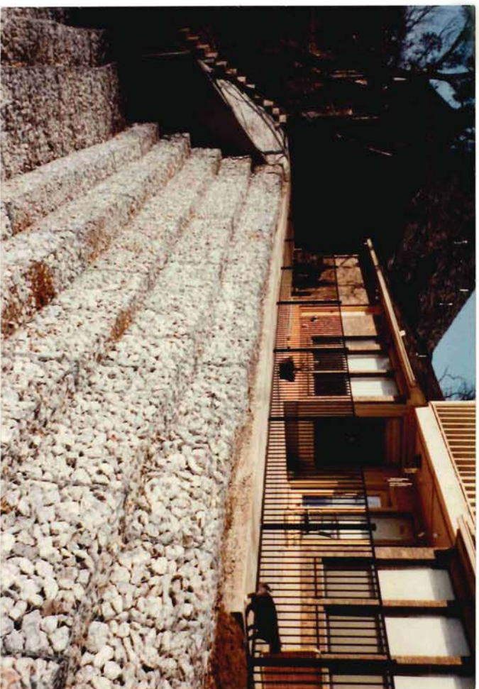
Photograph 6. Completed gabion section prior to 1991 flood. Camera pointed west towards residential Lot A.
