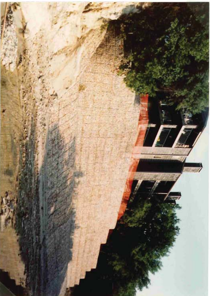
Photograph 2. Constructed thin section gabion wall with rock anchors. Construction cost $300.000.
