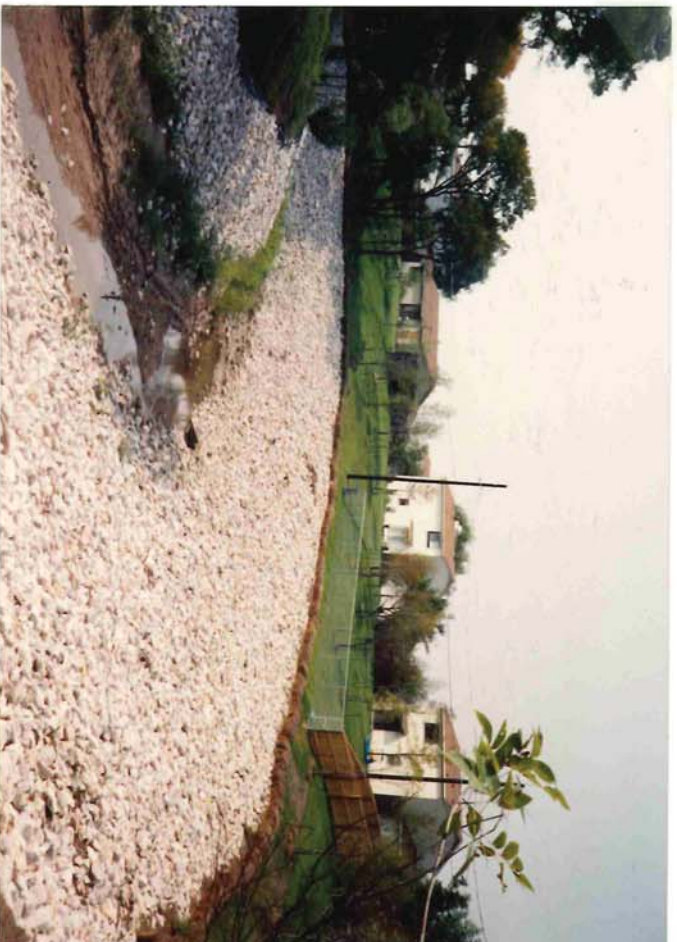
Photograph 13. Completed section of re-graded creek and armored slope. Residences at 417 and 413 Brandon Street in the middle and right of photograph.
