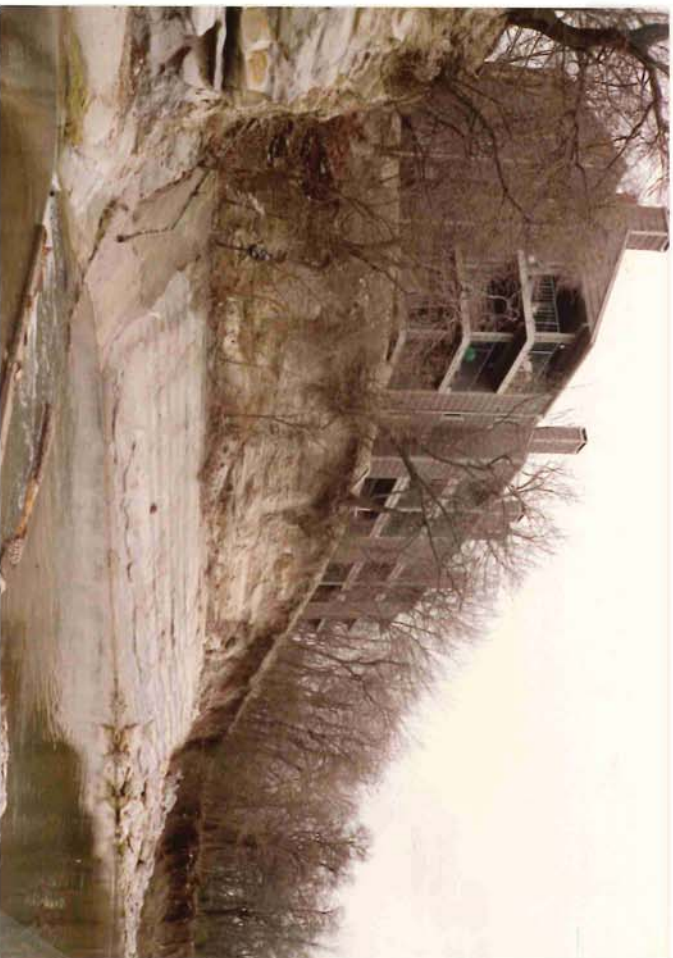
Photograph 1. Erosion and steepening of a cut bank within the Austin Chalk Formation. Note undermining of front corner of foundation.
