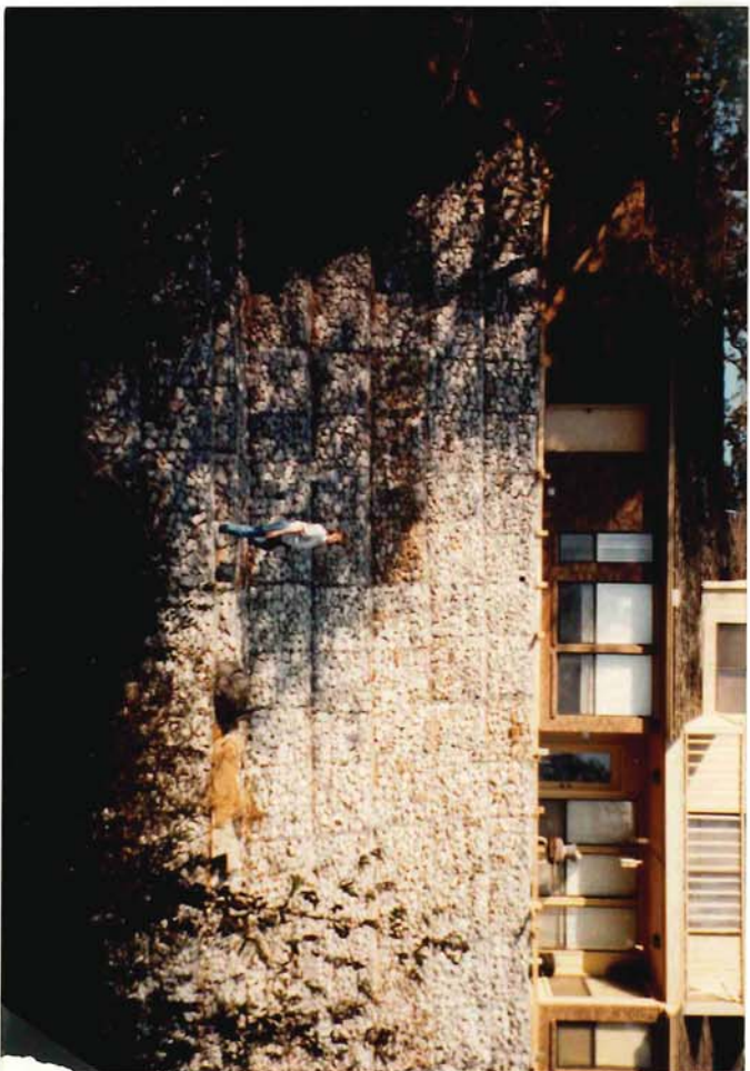
Photograph 5. Completed gabion section prior to November 1991 flood.
